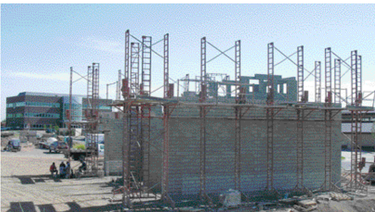
Block overruns were used in this project to save construction material costs.
