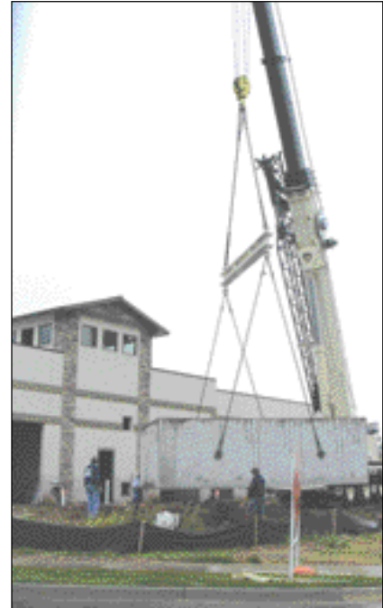
The installation of a 10,000 gallon water storage tank saved more than $100,000 in water tap fees on this project.
