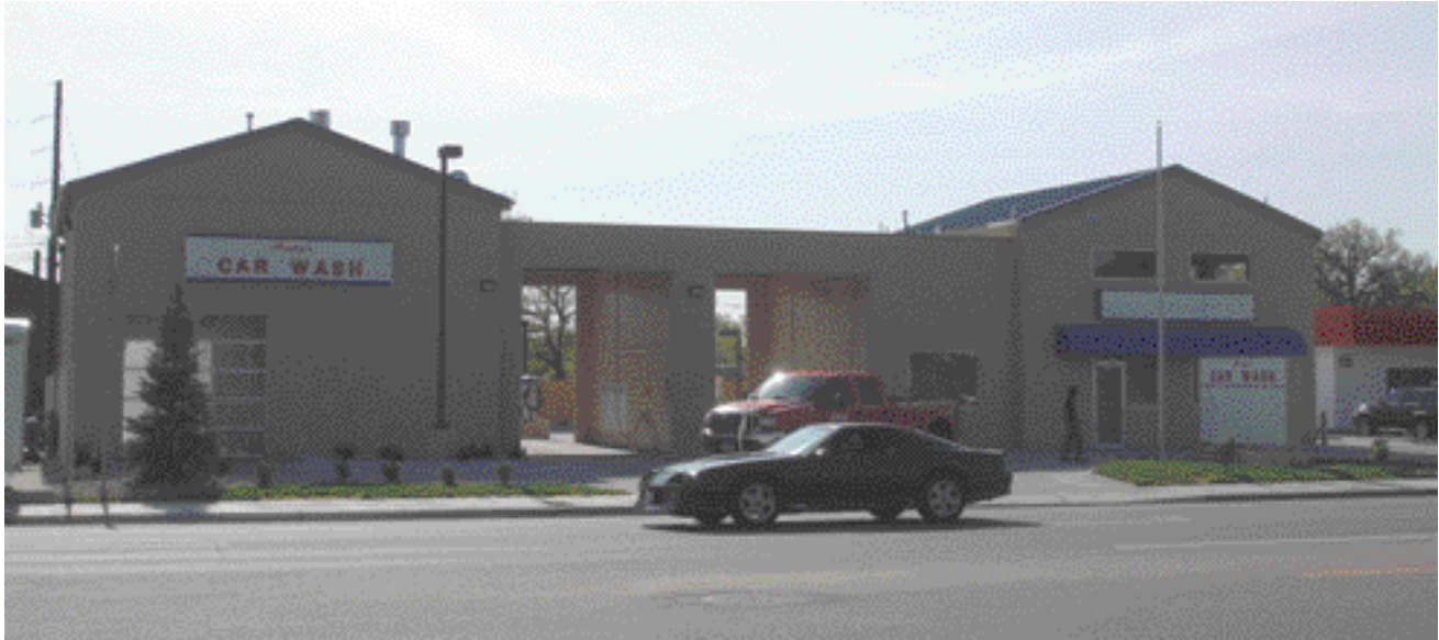
After: The new state-of-the-art wash features one automatic and two self-serve bays, with a connecting retail store and office above.
